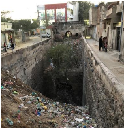
Fig -17: Present condition of Bawdi in Jhunjhunu (Source: Author)
