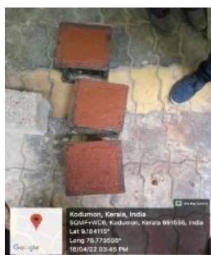
Fig -10: Casting of ferrock concrete
