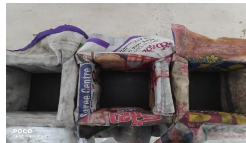
Fig.5 controlled permeable formwork
