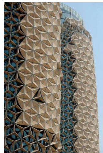
Fig -11: External Automated Shading System of Al Bahr Towers
