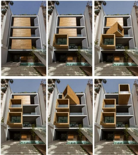
Fig -6: Sharifi-ha House in various stages of 'open' and 'closed' modes
