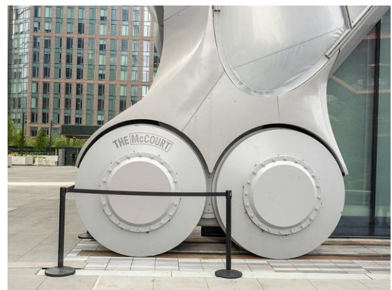
Fig -22: Wheels used to retract or extend the steel shell
