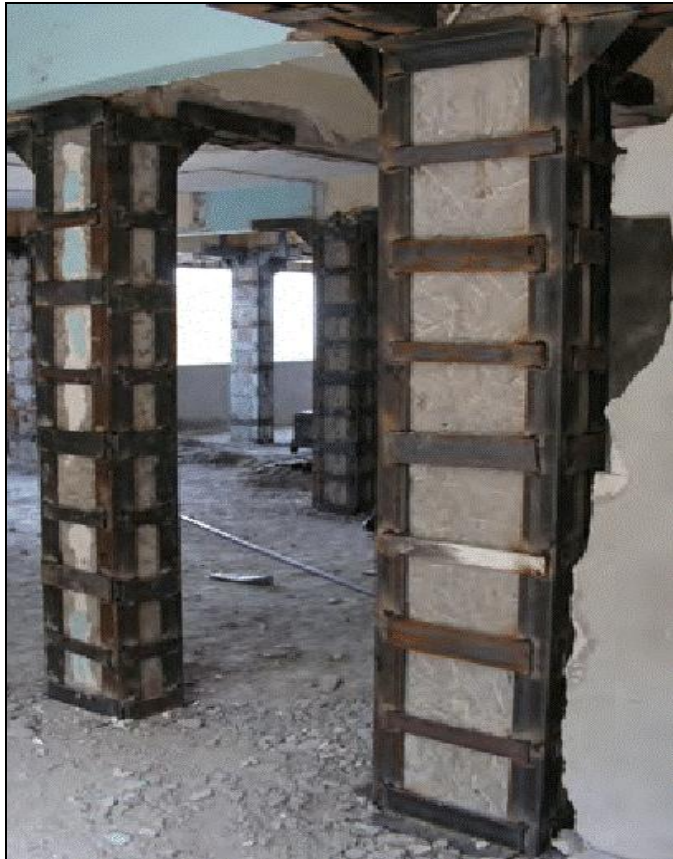
Fig. -4: Steel caging
