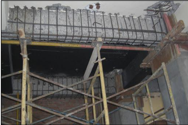
Fig -1: Concrete Jacketing
