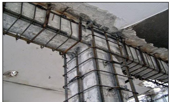
Fig -3: Steel Jacketing
