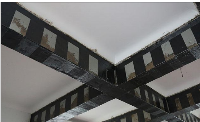
Fig -2: CFRP Jacketing
