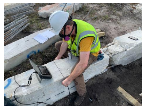
Fig -4: An engineer performing UPV test on a column member.
