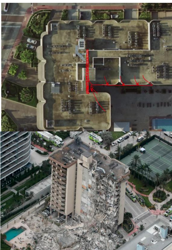
Fig -22: The shear wall is shaded in red colour in the right picture, the left picture shows the aerial view of the shear wall.
