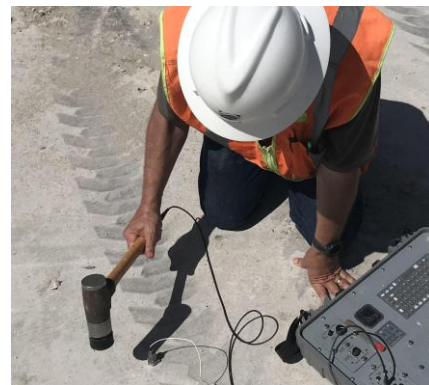
Fig -3: A geophysics specialist performs non-destructive testing, using an impulse echo, to support the evaluation of the integrity of the foundation.
