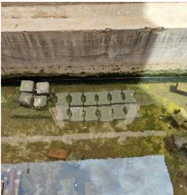
Fig 4 curing of paver blocks
