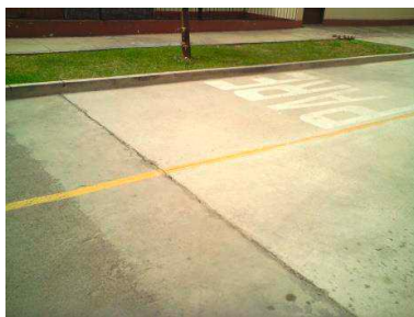
Photo 3.- Data in concrete surface.
