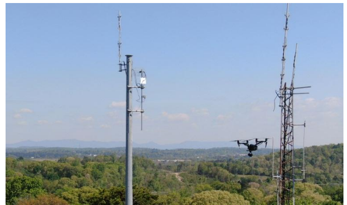
Fig. 10. UAS (drone) being used to confirm antenna alignment on Site B's radio towers (~85m height).
