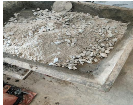
Fig – 3. Preparation of concrete mix
