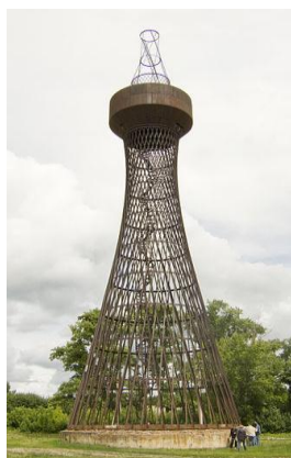
Fig -1.2: First Diagrid Hyperboloid Structure
