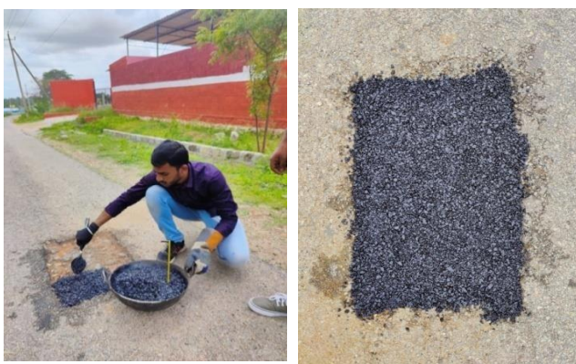
Fig-11: Bituminous Concrete Mix Laying
