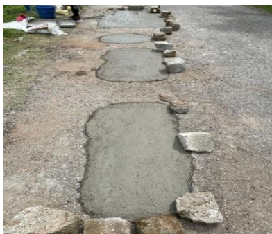
Fig-10: White Topping Laying
