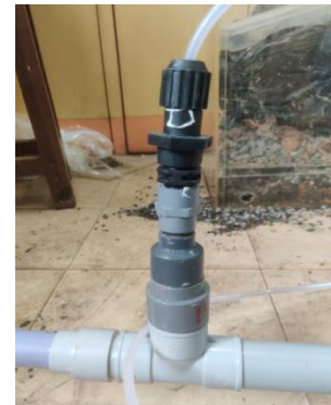
Fig - 8: Point of Chlorination
