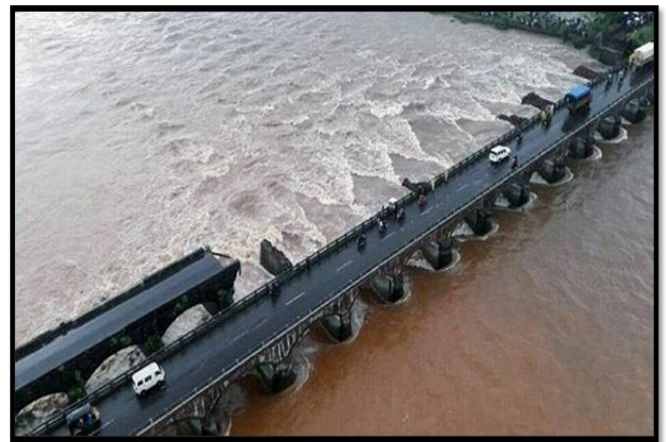
Fig -1: Bridge Failure
