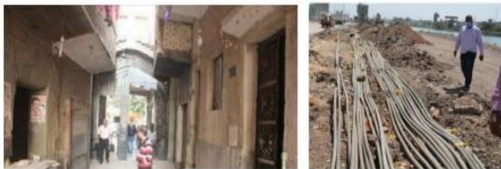
Figure 9: crumbling brickwork, and empty buildings
