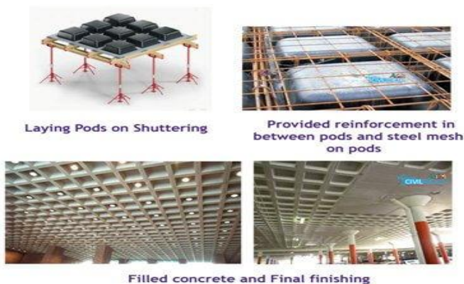
Fig -3: Waffle Slab
