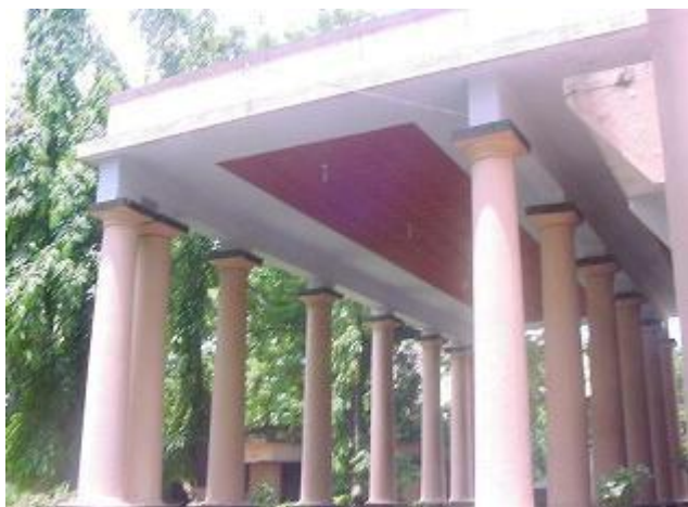
FIG 7 .AFTER THE CONSTRUCTION COMPLETION
