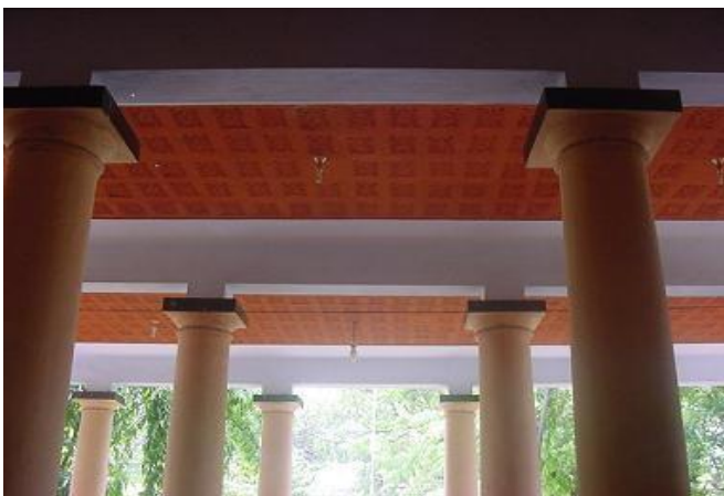
FIG 6 .AFTER THE CONSTRUCTION COMPLETION
