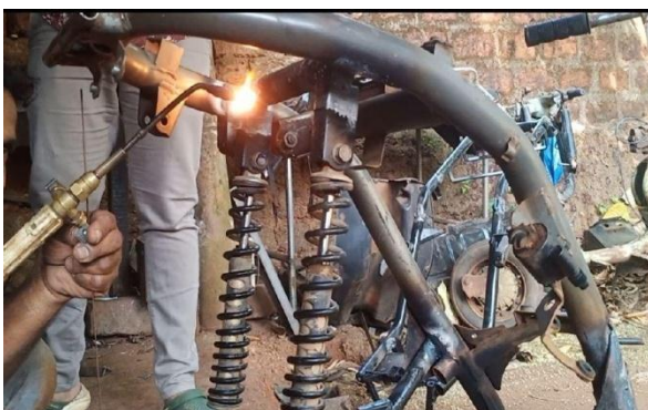
Fig 4: Fixing the new suspension system
