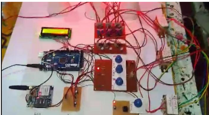
Fig -3: Working model of IOT based fault monitoring system of three-phase
