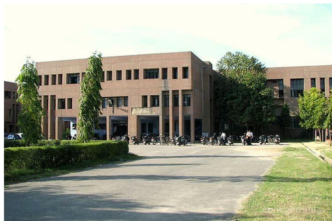
Figure1. Flexible Pavement at IET Lucknow
