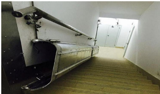
Figure 3: Combined stair and slide way evacuation
