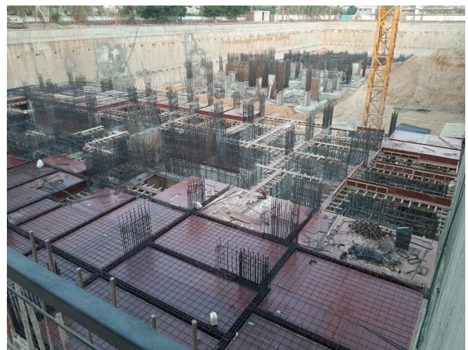
Figure 2- Site Photo Of Harmony Harikesh Apartments
