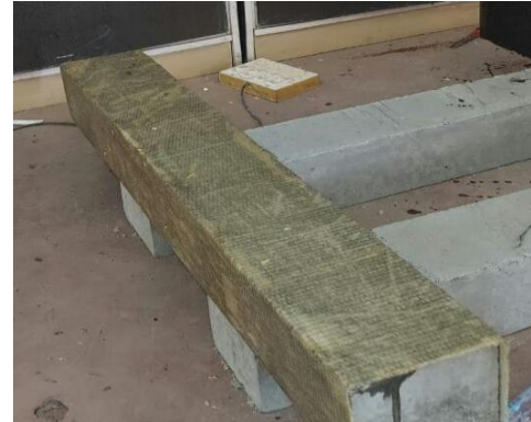
Fig.3: Retrofitting of beam using GFRP
