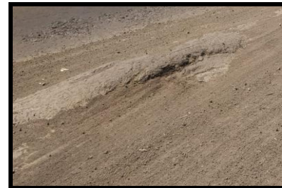
Fig 5 : Slippage cracks
