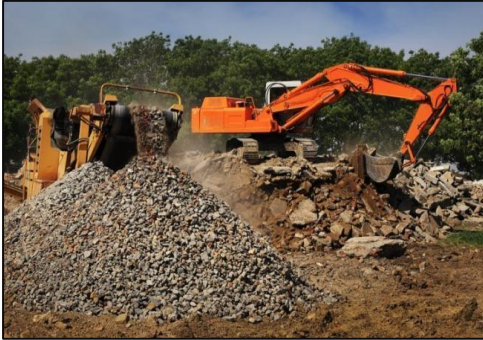
Fig. 1. Demolished Concrete Aggregate
