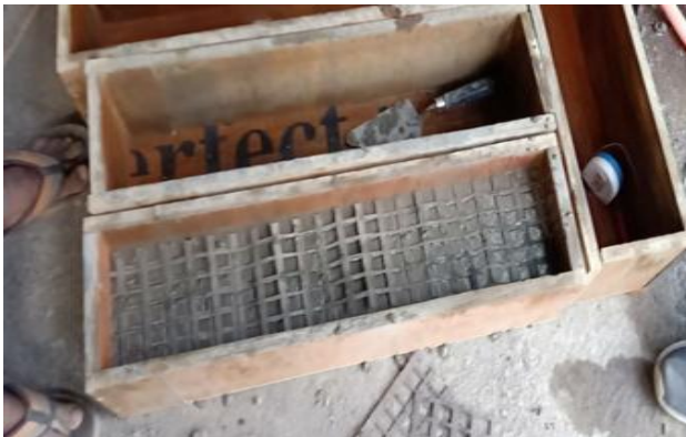
Fig.3 Placing of Geogrid.
