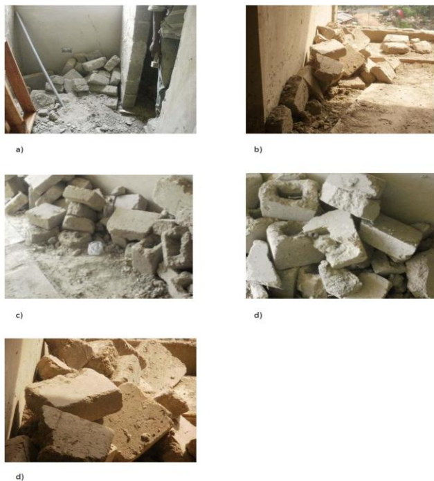
Fig 3. Wasted cement/mortar on construction site
