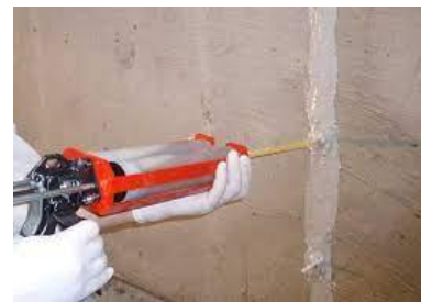
Fig-6: Epoxy are filling in crack.
