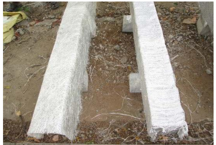
Fig-6: GFRP Wrapped Beam - 400GSM
