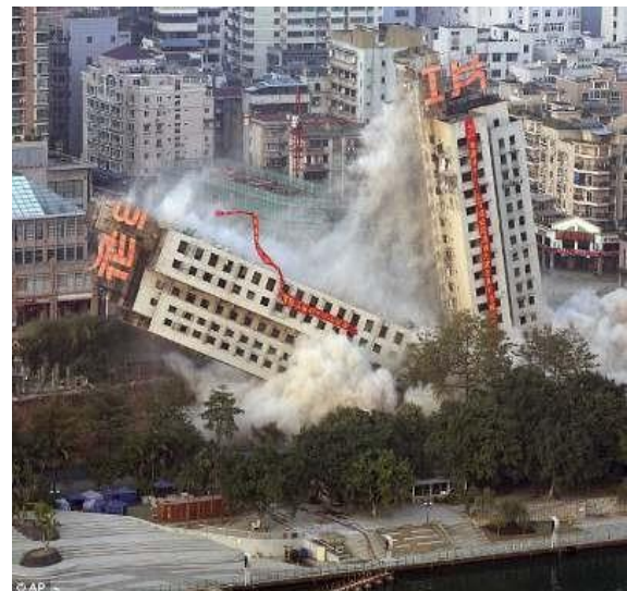
Fig -1: Splitting of a tall structure into two portions in a vertical manner at Oogue at Siberia
