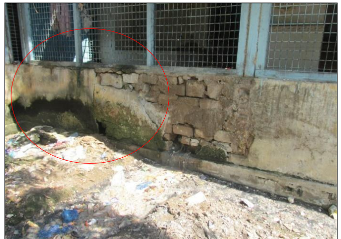
Fig -2: Loosening of Motor
