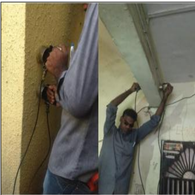
Fig -7: a) In-situ Non-destructive Tests
