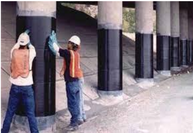
Fig -2: FRP wrapping on column
