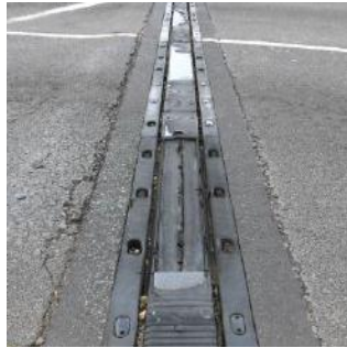
Fig -16: Breaking up of materials from the expansion joint
