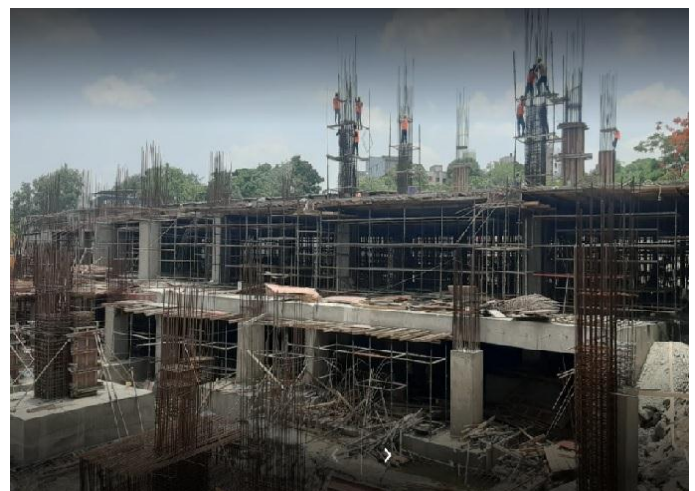
Fig-2 : Construction work of Le Skylark Project
