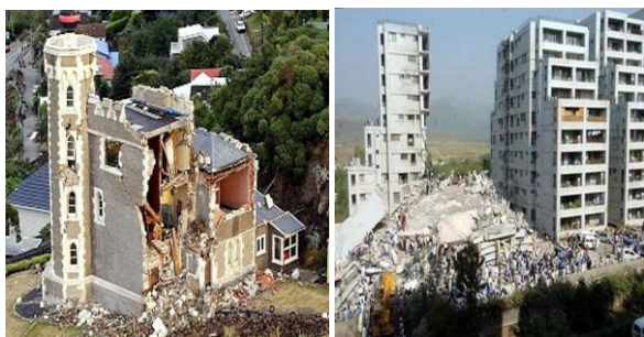
Figure 5 Behaviour of Stepped building in Earthquake
