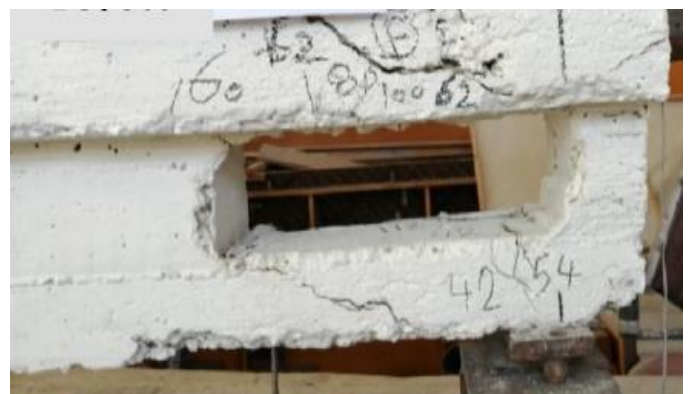
Fig-6: Failure mode of flanged deep beam
