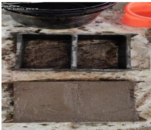
Placing of mixed materials in mould
