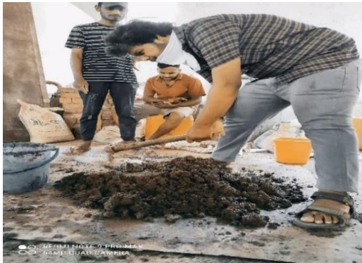
Dry mixing of materials
