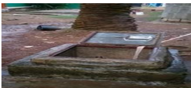
Figure 4 Shallow Hand Dug well
