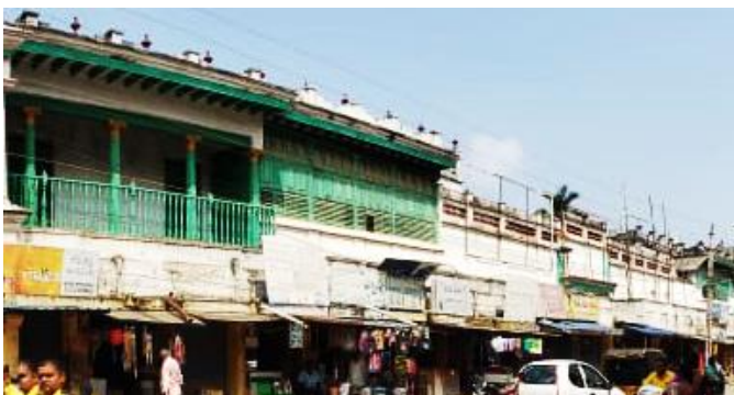
Fig -7: Timber work on North- Eastern wing
