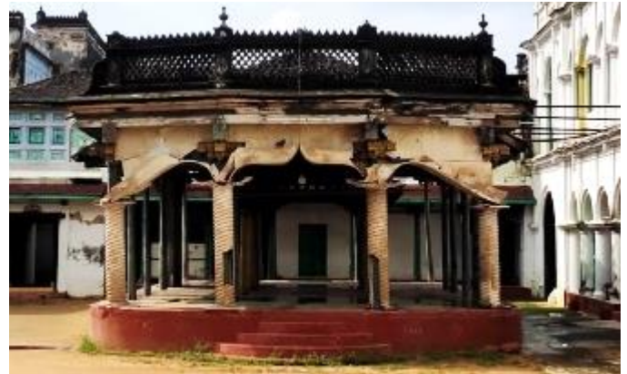
Fig -8: The front view of pillared platform
