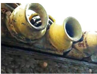
Fig -10: The pots used as gutter; Fig -11: view of the room.
