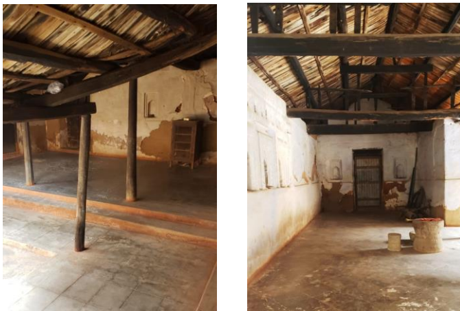
Fig-1: The roof lowered at the center providing shade.
