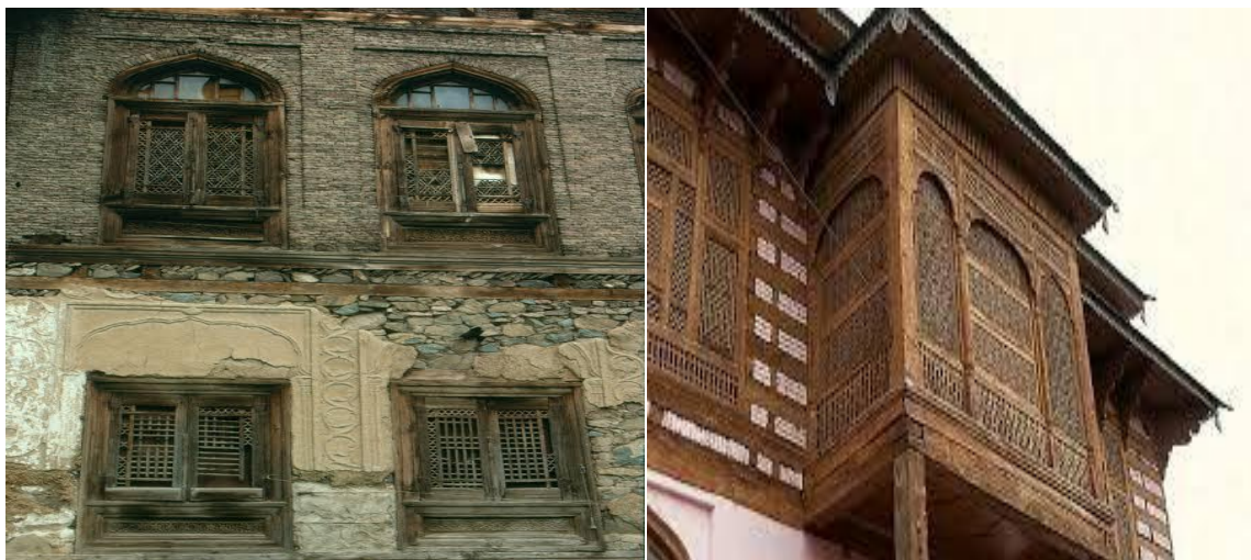
Figure 2 and 3 : panelled windows
