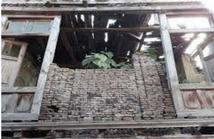
Figure 4: maharaja brick wall
