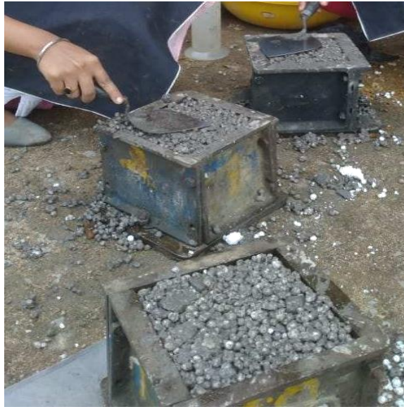
Fig 2.2: Mixing of cement, sand and aggregate with water.
