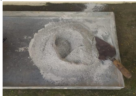
Fig -1: Mixing of materials
