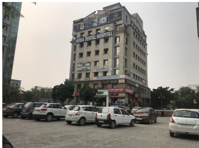
Figure 16. Sunrise Tower (Source: Field Work, 2020)
