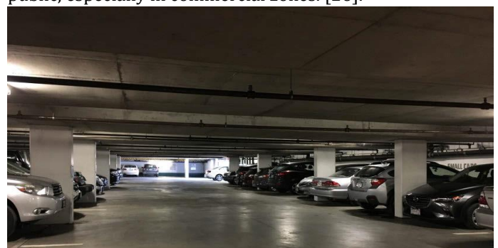
Figure 4. Underground parking lot [27]
