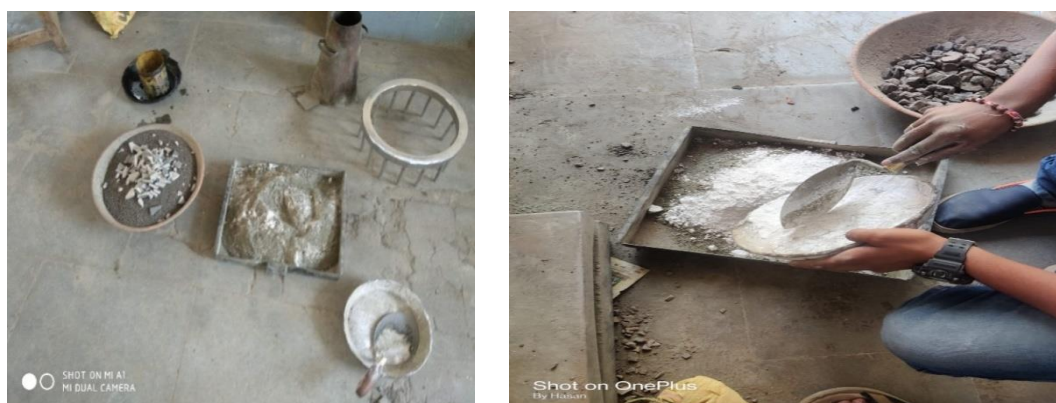
Fig 2: preparing of dry mix
