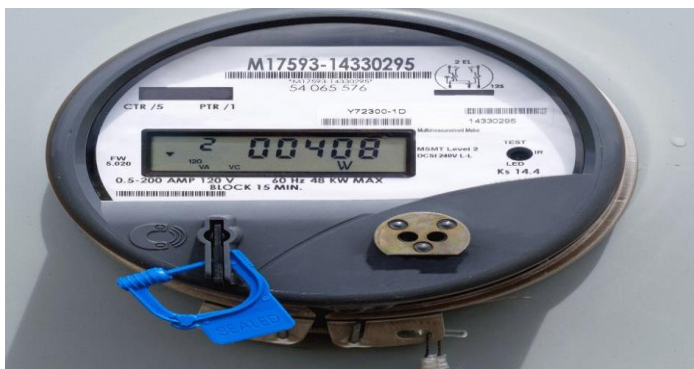
Fig-1: Net Energy Meter
