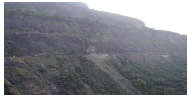
Figure 13. Case 3 Typical locations on existing road where RCC Retaining wall can be proposed.
