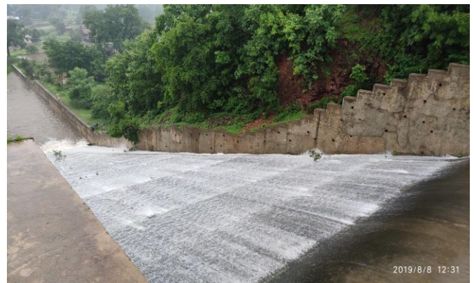
Figure 1 Spillway functioning in Monsoon
