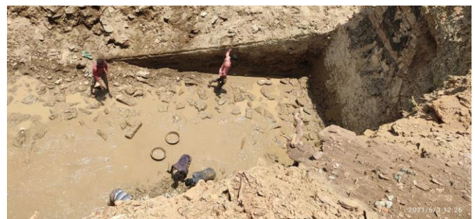
Figure 5 Dumping of rubbles manually
