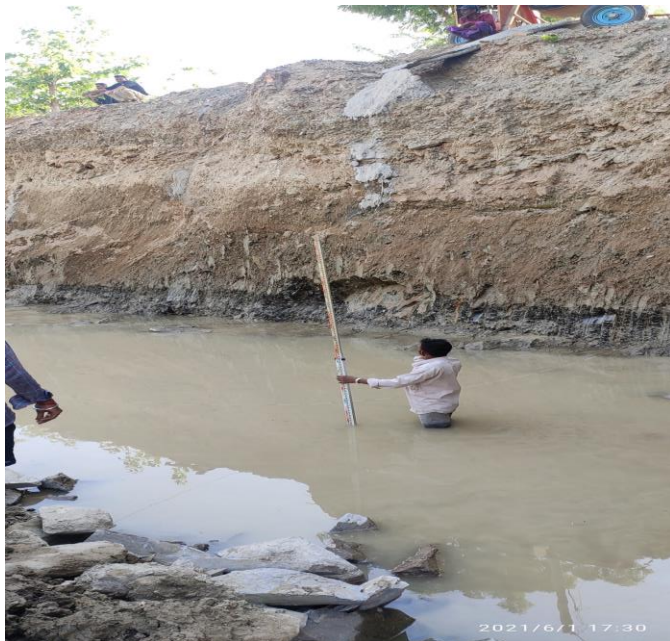
Figure 3 Knee height water after 15 minutes of dewatering
