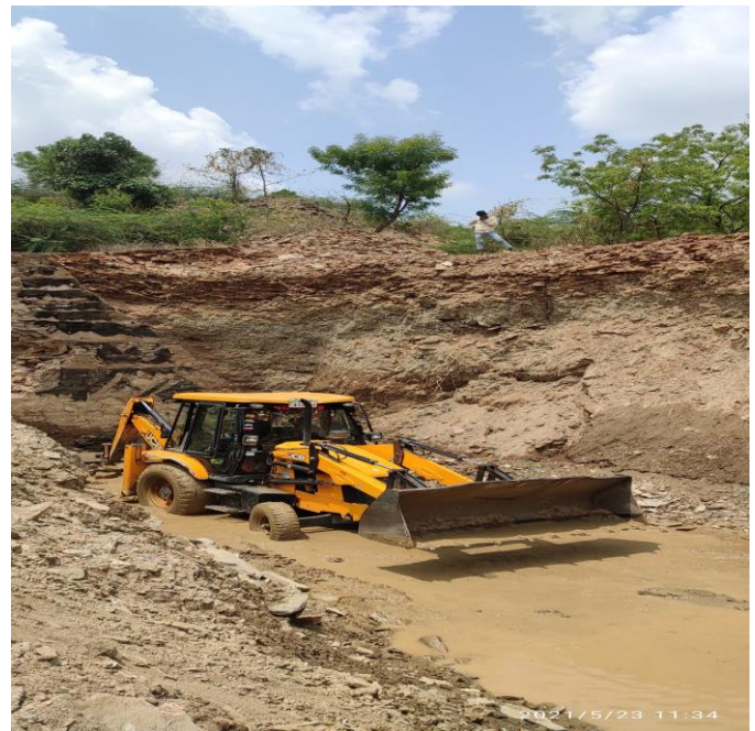
Figure 4 Removal of the muck after initial dewatering
