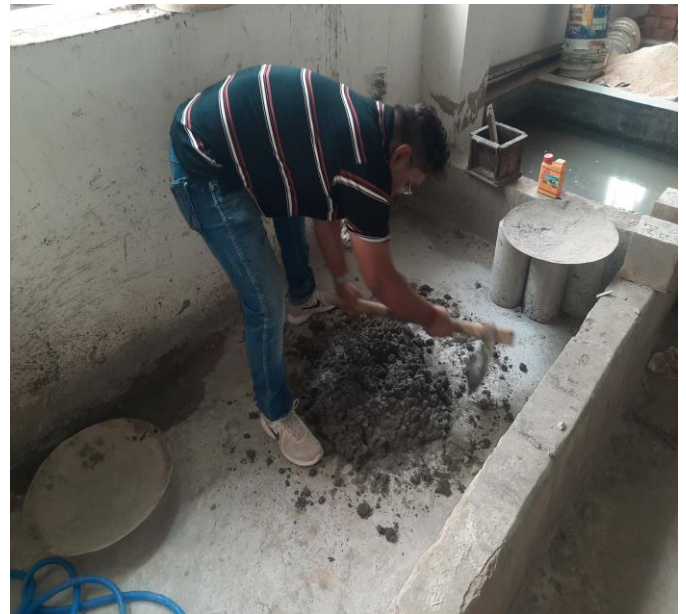
Figure 3.0: Process of Hand Mixing of Concrete
