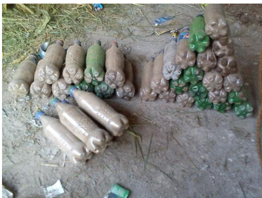
Fig -1: Filled plastic bottles with sand
