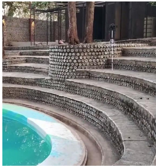
Fig -5: Plastic bottle wall construction for swimming pool and steps, garden
