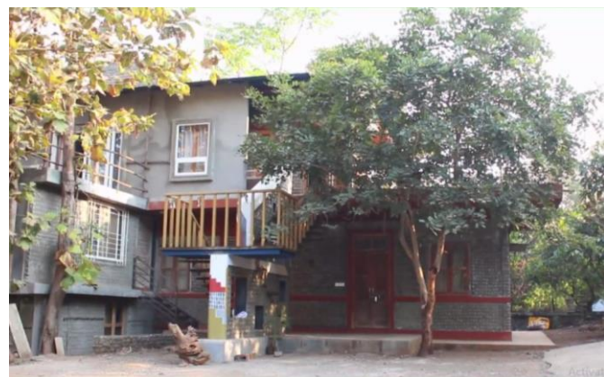
Fig -4: Plastic bottle wall constructed bungalow
