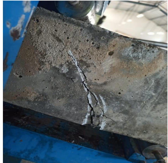
Fig -4: crack pattern of beam with steel fibre on tension zone
