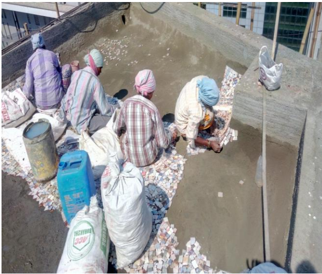
Fig -6: Fitting China Mosaic chips
