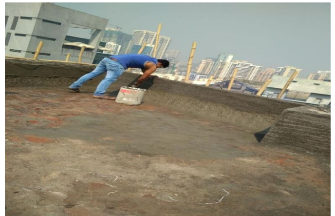
Fig -4: Applying coating
