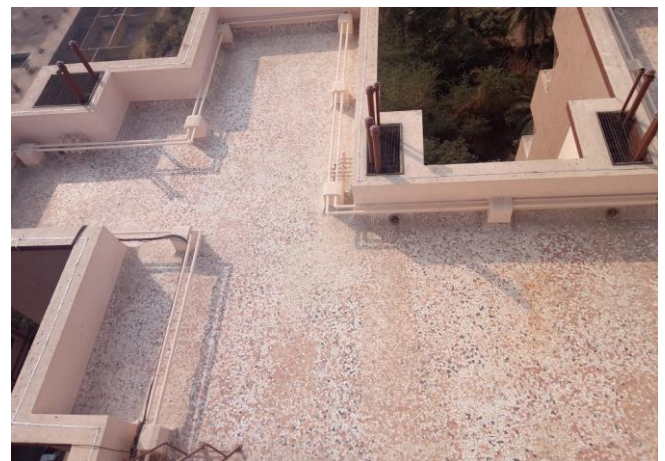
Fig -8: Finished Surface
