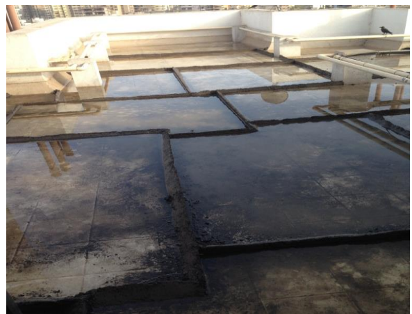
Fig -1: Water ponding Test
