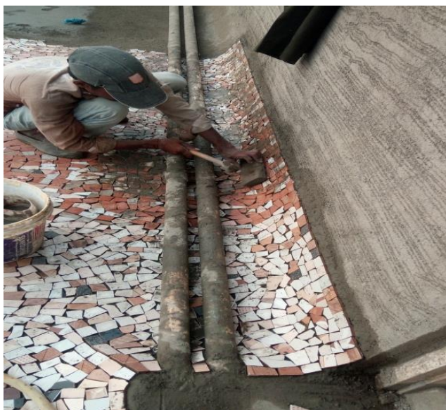
Fig -7: Pressing CM chips with Mallet
