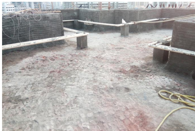
Fig -3: After Breaking of IPS
