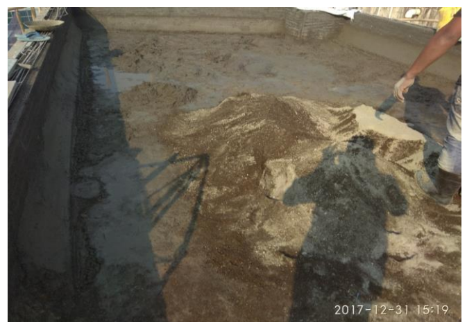
Fig -6: Spreading Cement-Mortar
